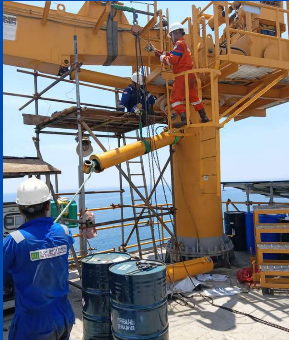
PERTAMINA HULU ENAERGI WMO CW PLATFORM Luffing Cylinder Replacement
