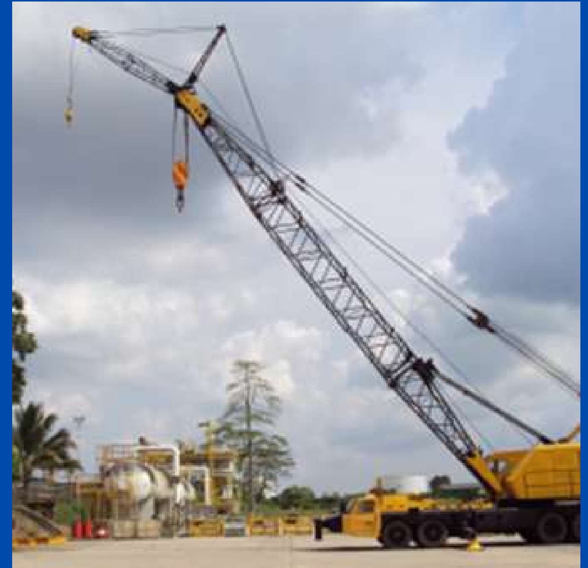
Attaka Field-NIB Serang-Sepingga Yakin-Santan & Lawe2 terminal 34 Units Offshore & Onshore Crane Preventive Maintenance & Service Contract (3years) - Chevron Indonesia Company
