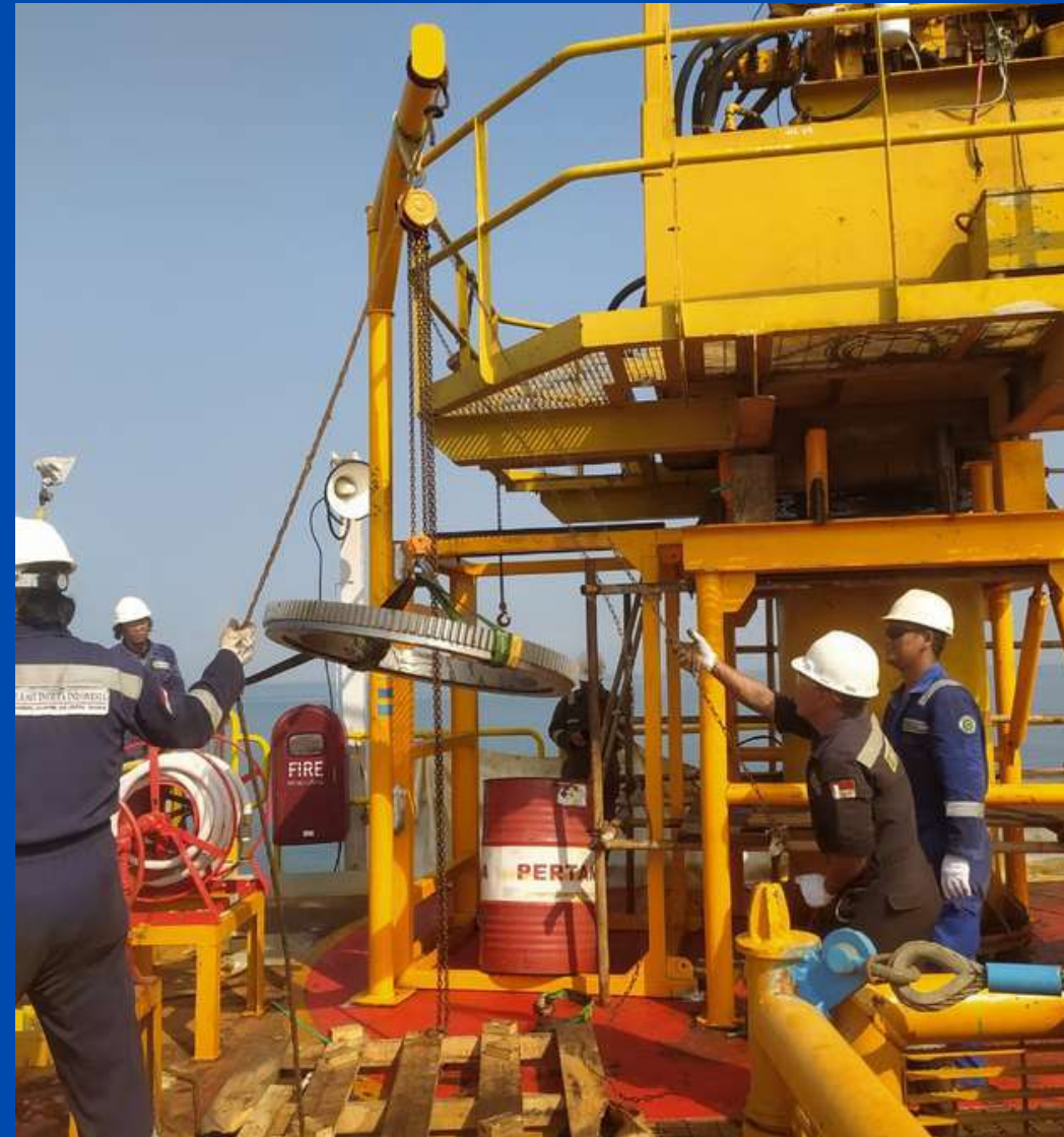
Attaka Field - Satelite Platform Pertamina Hulu Kalimantan Timur slew Bearing Replacement
