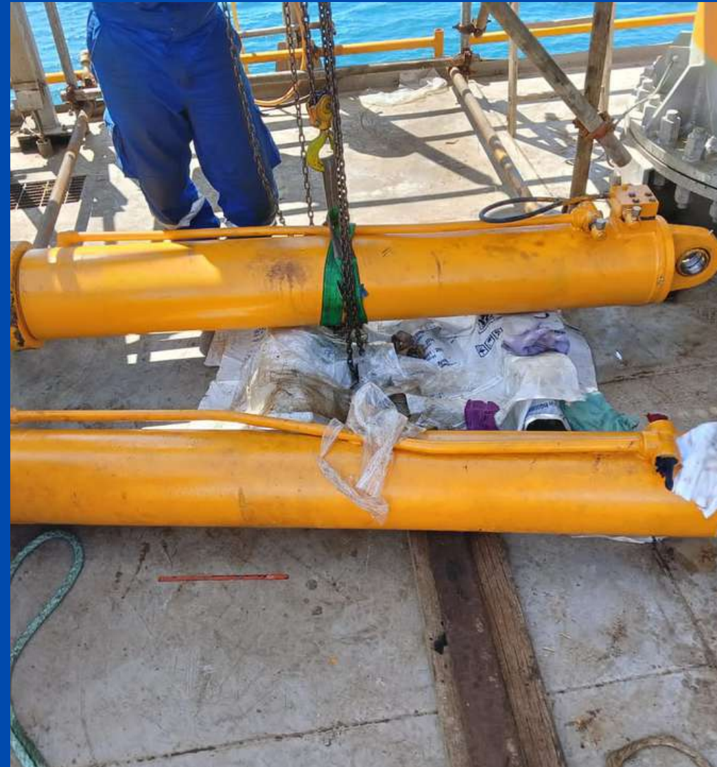
PERTAMINA HULU ENAERGI WMO CW PLATFORM Luffing Cylinder Replacement
