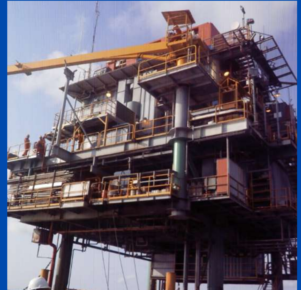
PERTAMINA HULU ENAERGI WMO 15 Units Offshore & 1 unit Onshore Crane Preventive Maintenance & Repair Service
